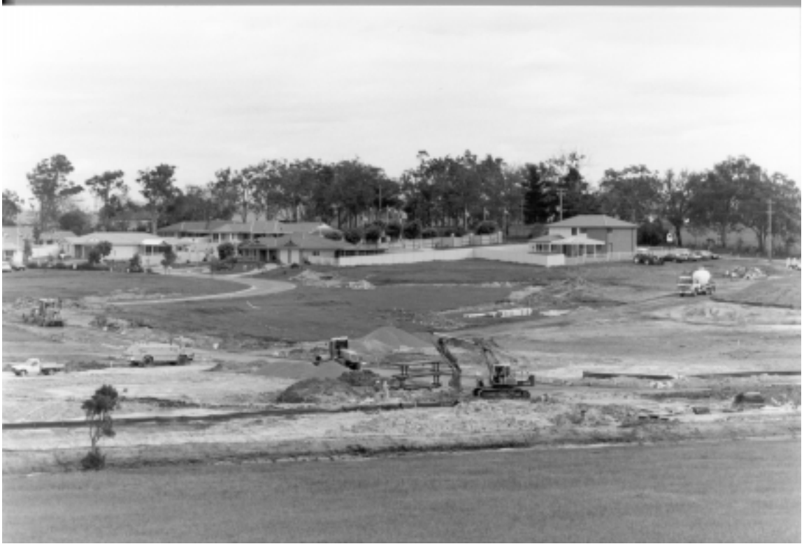
Residential Development along the Wallarah Road, near Kanwal, May 1998. Increased sediment loads in nearby creeks are often observed during the construction phase, due to removal of vegetation and disturbance of soil.
